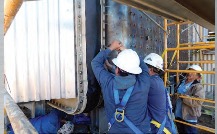
10' x 15' X 12" face-to-face fabric expansion joint belt and bolster replacement in a Louisiana gas turbine power plant
