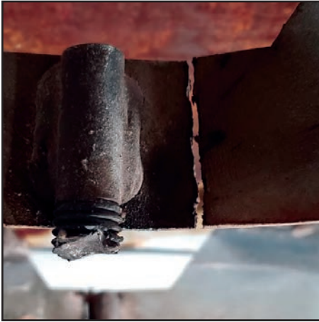
Typical scallop bar crack
