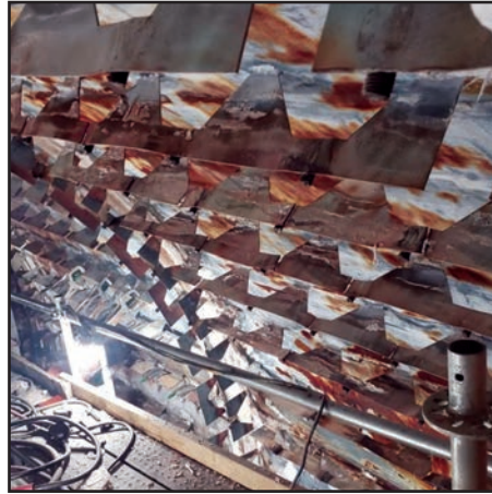
Scallop bar distortion and cracks
