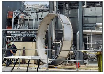
147" diameter Alloy 625 Gr. 2 bellows with covers and liners installed on this large frame turbine exhaust joint
