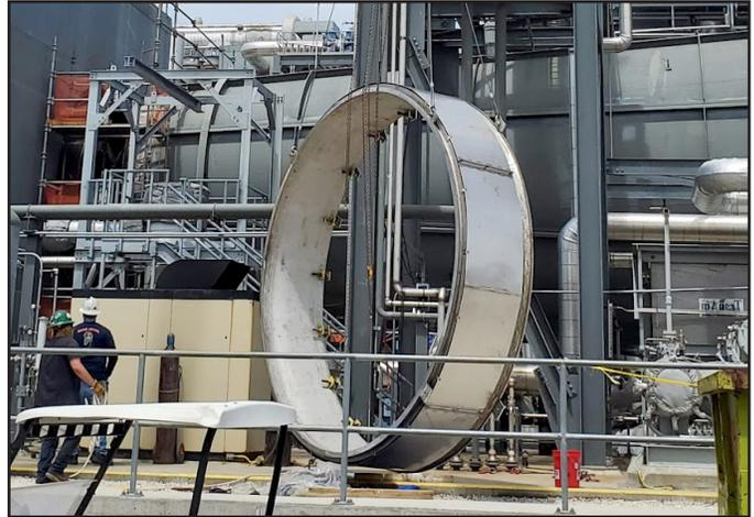
147" diameter Alloy 625 Gr. 2 bellows with covers and liners installed on this large frame turbine exhaust joint
