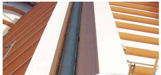
Fabric material selection is key to ensure the expansion joint can withstand the corrosive environment
